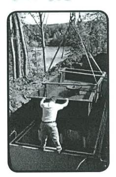
Bio-Microbics FAST® wastewater treatment systems provide alternative options for properties residing outside the reach of municipal (public) treatment plants. FAST® systems can be used for new construction or retrofit in existing tanks; including those in nitrogen sensitive areas or limitations with distance to groundwater and/or smaller dispersal field size requirements. Engineered to fit most typical residential and commercial applications.
